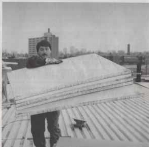
A roofer demonstrates Perma-Therm's light-weight characteristics.
