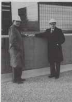
A Perma-Seal-capped parapet wall is seen behind FCI reps Jim Turnbull, left, and Paul Davis.
