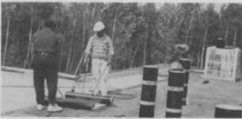
Two-ply Perma-Seal roof membrane being torch applied.
